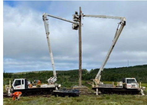
Single pole construction on transmission line 94L.
